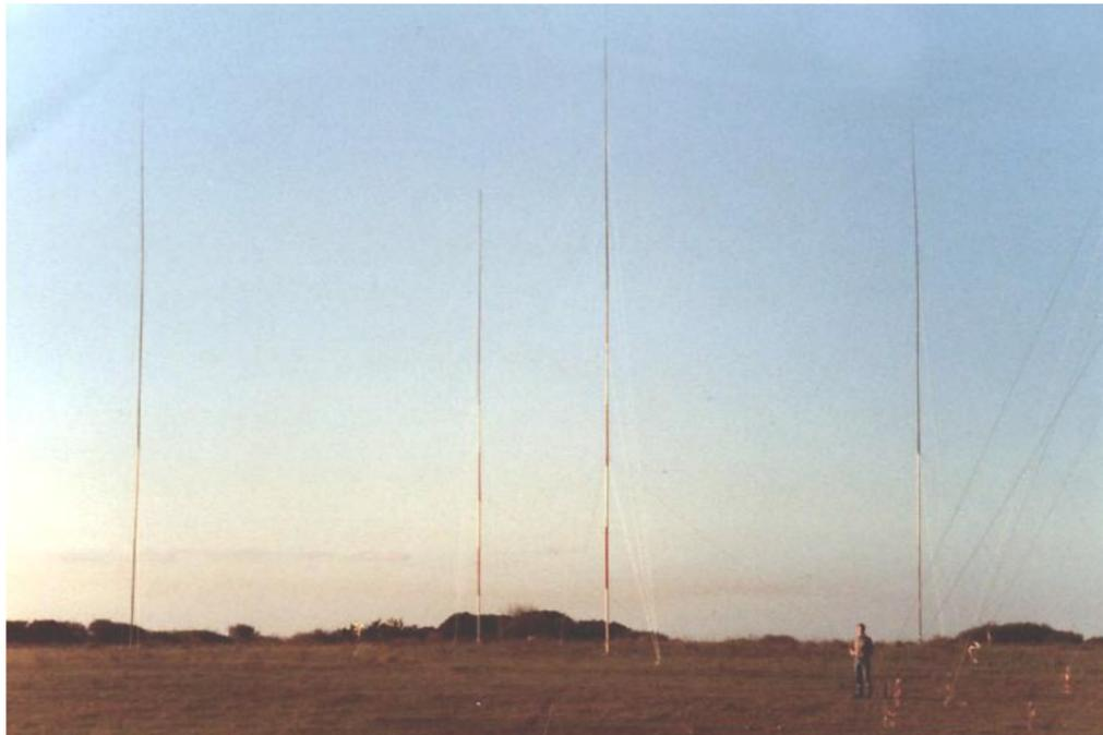
This page is a short description of the four phased verticals system i've build and used. It is primarily intendend to be used on the lower bands 160m, 80m, 40m. All the principles stated here are of course valid for any other bands, but you can achieve the same game with yagi antennas easily. It is mainly built around the Collins hybrid phasing system wound on toroids.
